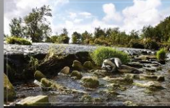
WEIR Ort: Gronau Location: Leine-Wehr Model: Alexandra
